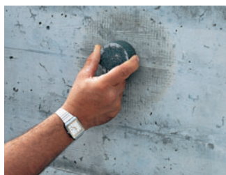
Smoothen test area with a grinding stone.
